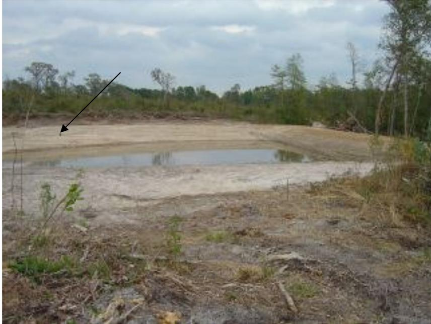
The arrow indicates the height of the spill/drain pipe. To its left is an emergency spillway should the water rise too fast. The drain pipe will be the water height of the pond.
