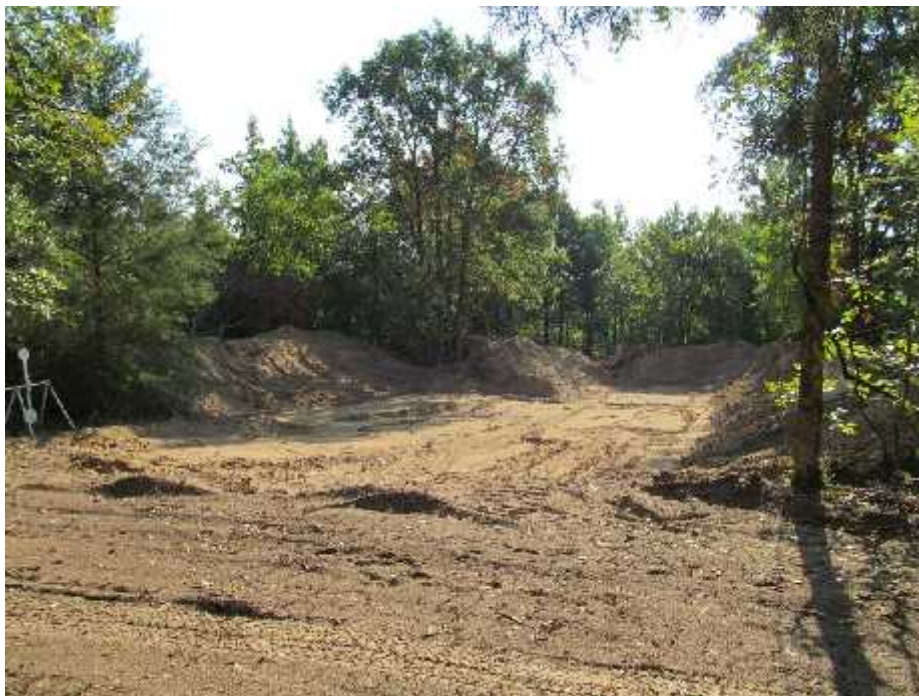
This is the foot print of the new 7 room shoot house.
